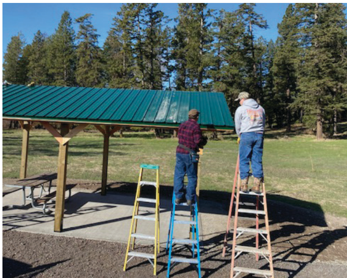
Volunteers from Flathead Wildlife, Inc. construct the picnic shelter at Pine Grove Pond Fishing Access Site. Photo courtesy of Jim Vashro.
